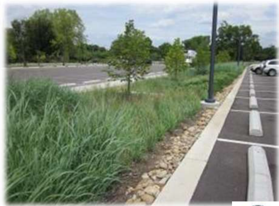
Parthenon Parking Lot Bioretention Basin
