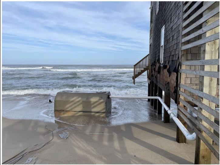
An exposed septic tank on the Cape Hatteras National Seashore in Rodanthe. Photo: National Park Service
