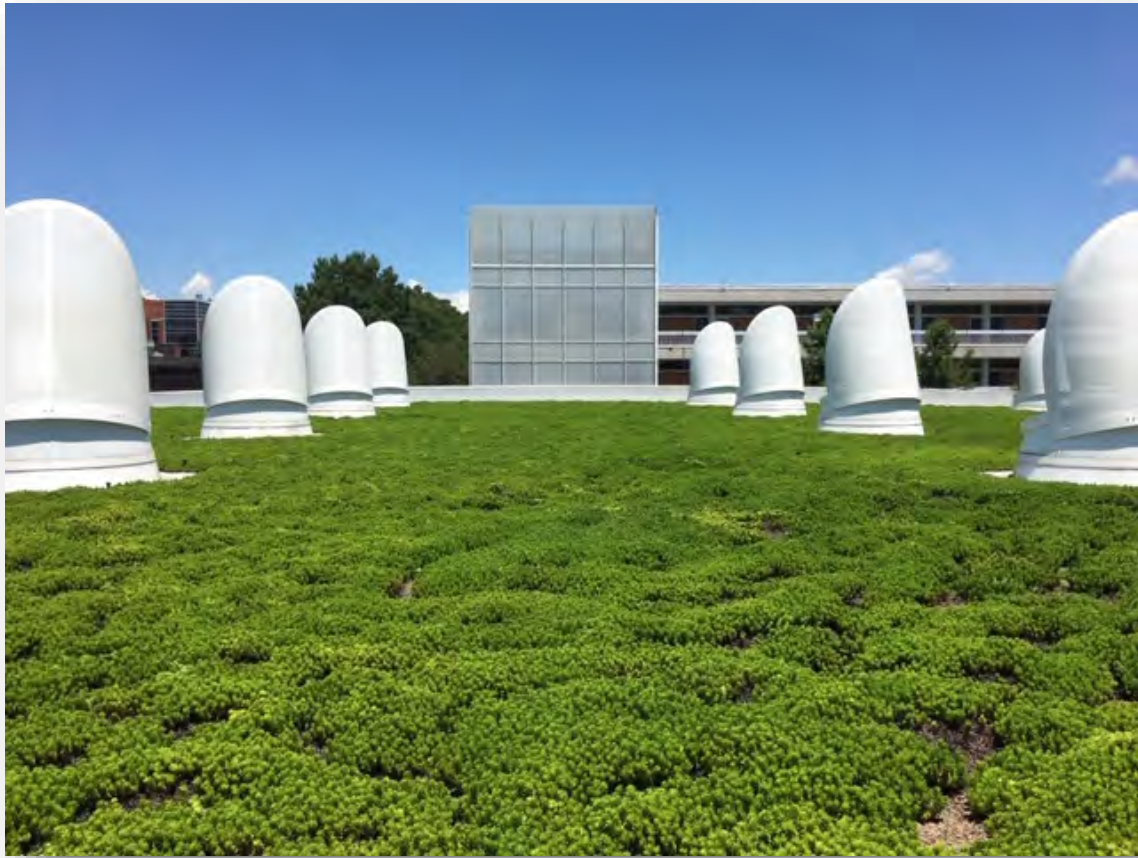
Lee Hall Green Roof
