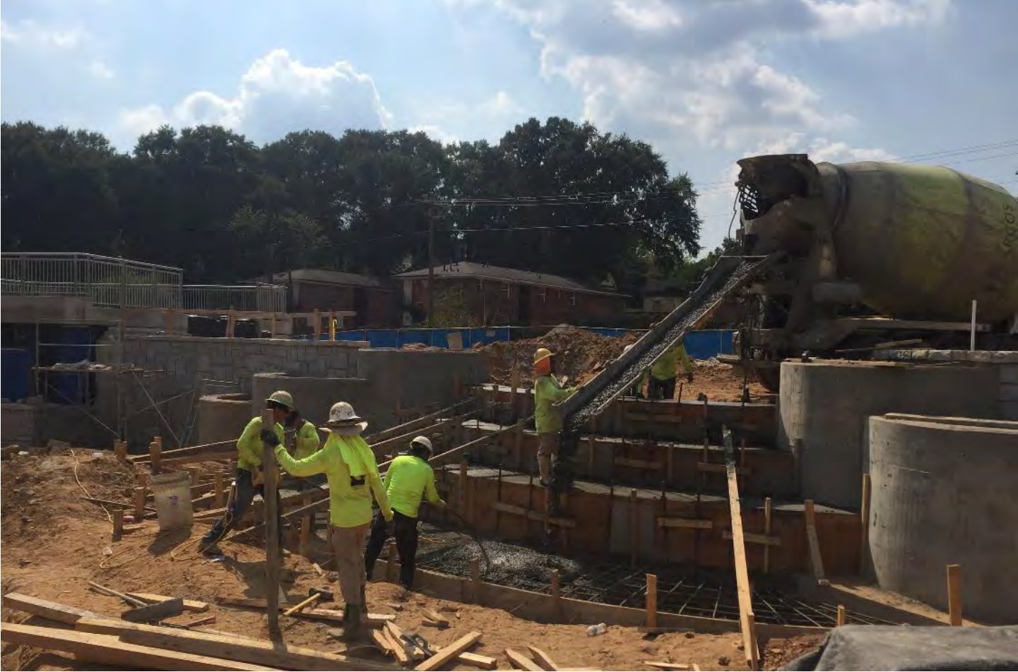
Cook Park – Restroom building / retaining walls near splash pad October 1, 2019
