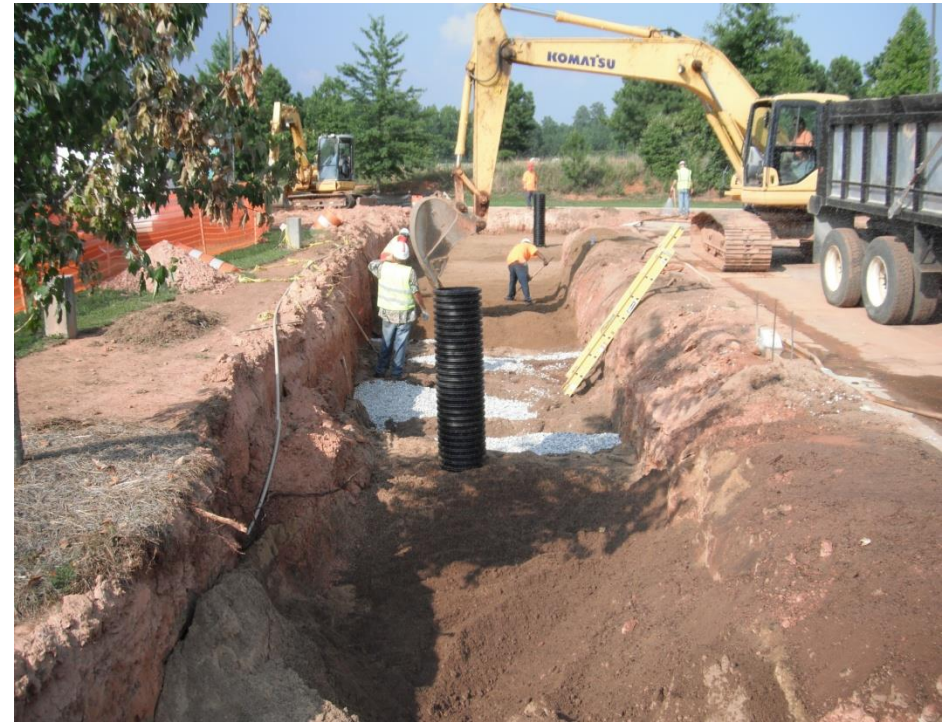
Installed gravel trenches across area to aid in runoff distribution.
