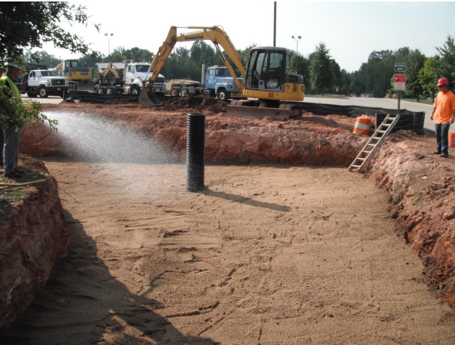
Installed engineer soils in 1 ft lifts and watered to consolidate.
