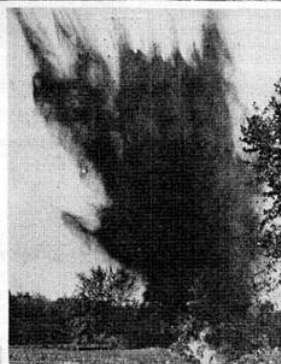
Straightening of Pequest River in New Jersey by CCC workers stopped its yearly floods. Location of new channel is seen at right. Note temporary dam at left to provide volume of water for scouring blasted channel.
