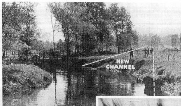
Straightening of Pequest River in New Jersey by CCC workers stopped its yearly floods. Location of new channel is seen at right. Note temporary dam at left to provide volume of water for scouring blasted channel.
