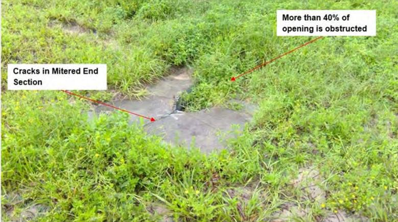
Cracks in Mitered End Section
