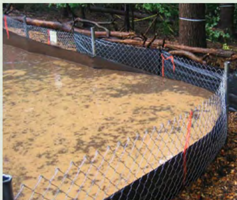
Construction Site Runoff Control Minimum Control Measure
