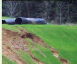
The slope of this berm has failed and eroded, requiring regrading and replanting
