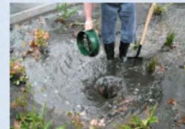
The outlet screen was filled with debris. After removal and cleaning, water can flow again
