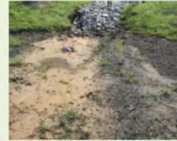
Sediment has accumulated in the infiltration area and needs to be cleaned out. Clogged media may require replacement
