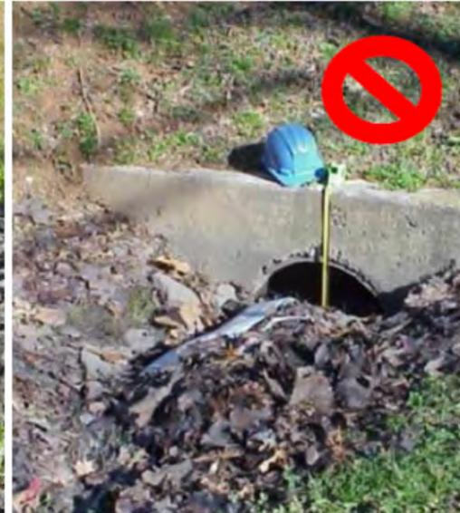
**Pretreatment** is the first layer of protection for the main treatment area. Debris and coarse sediment are removed, which reduces clogging in the main treatment area. The pretreatment area can be cleaned more easily than the main treatment area. It should be free of sediment, trash, and debris. Erosion, scour, and damage should be evaluated.
