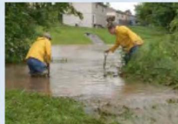
The outlet has clogged, which has led to flooding of the BMP and nearby property.
