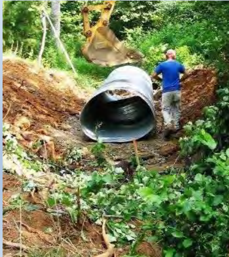
Culvert Replacement on UT Purlear Creek, Wilkes County, NC
