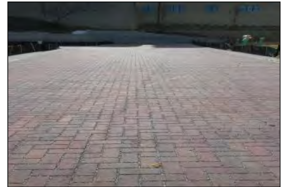
Permeable Pavers - Lakemoore Townhomes
