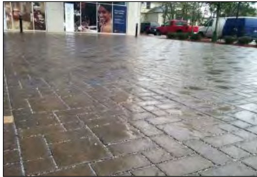
Permeable Pavers - 6 th and Juniper
