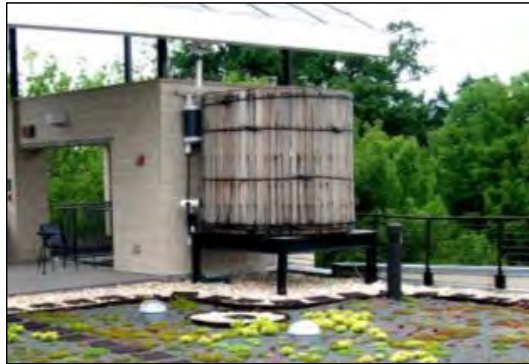
Cistern & Green Roof - Southface
