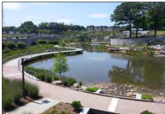
Wet pond, wetlands bench, sewer capacity relief, urban reforestation - Historic Fourth Ward
