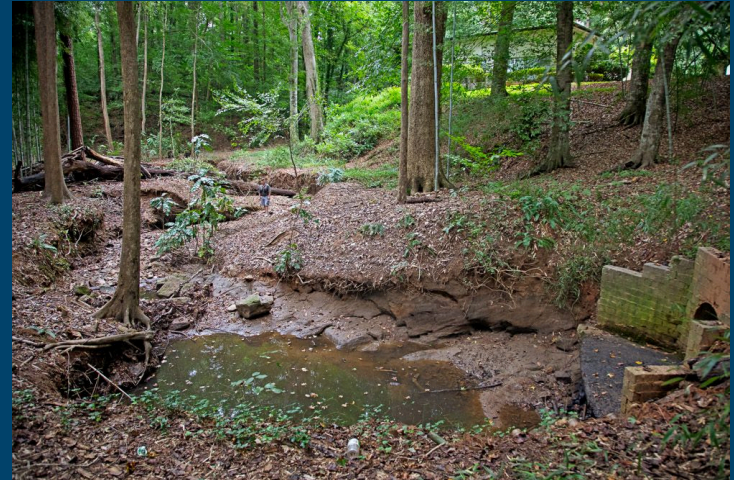
Minor-Moderate Erosion Stream Stabilization
