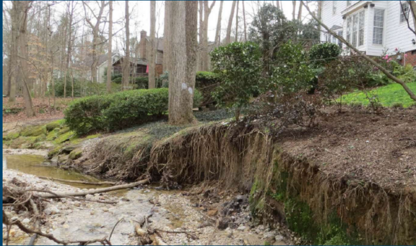
Major Erosion Drainage Assistance
