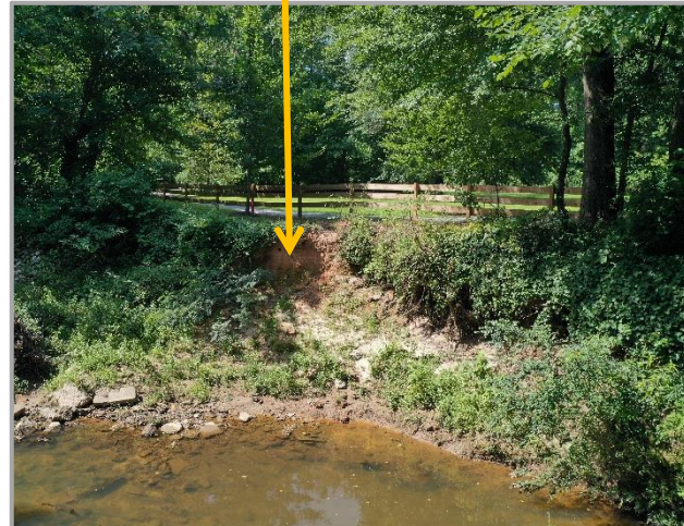
Bank erosion undermining fence (previously moved)
