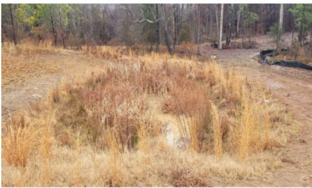
Existing conditions CP-SCM#6
